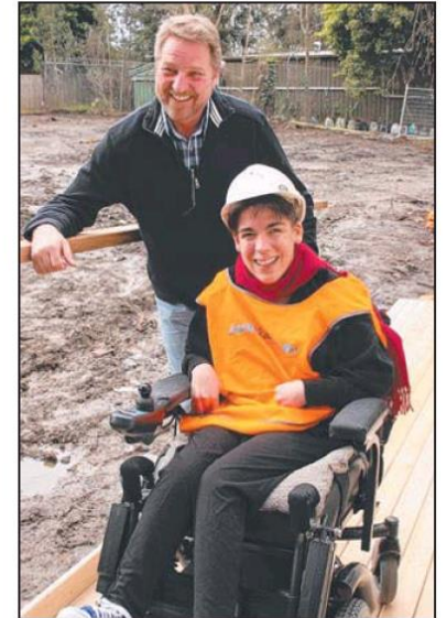
John Pendavingh, boss of builder Jorant Pty Ltd, and Caz Evans at EACH's new development. Picture: DANIEL MEREI
